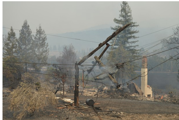
Shutting of Electrical Power during windstorms - $ ?
