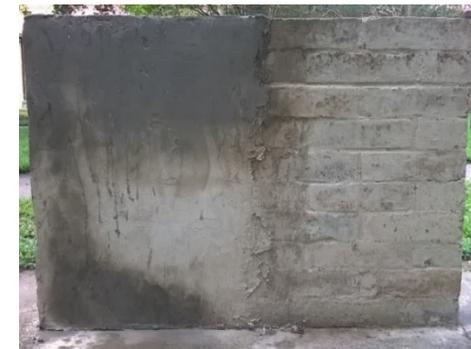
*Masonry wall after application of soil-cement mortar and cement paste*
