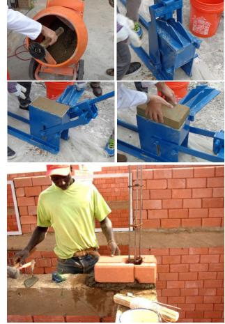
Masonry built using earth block fabricated by mechanically compressing a chemically stabilized soil mixture
