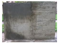
Masonry wall after application of soil-cement mortar
